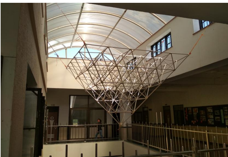
SPACEFRAME IN ARCHITECTURE DEPARTMENT MATERIAL – PVC PIPES
