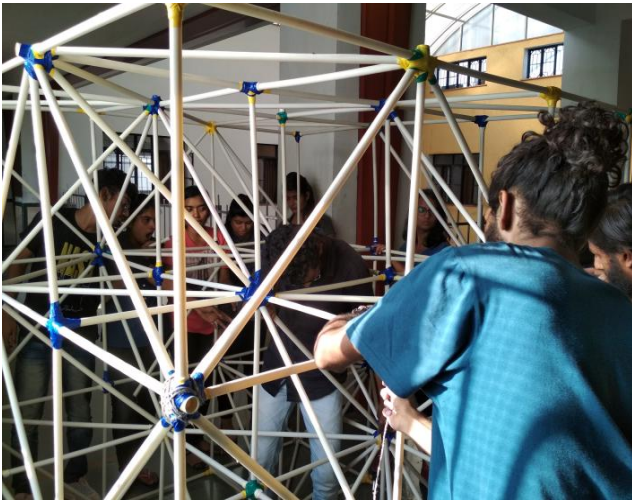
SPACEFRAME IN ARCHITECTURE DEPARTMENT MATERIAL – PVC PIPES
